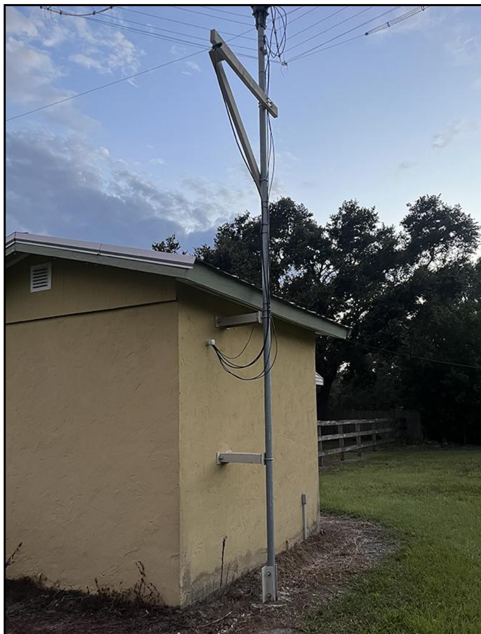
Photo 2: Close-up of mast with tilting base and supports (Photo: Dannette Herrmann)
