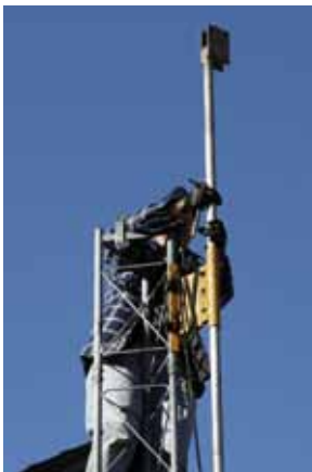
From left to right: KK1W attaching Gin Pole, securing foldover section; two views of 80 meter Double L antenna supported by tower; W1MJB looking on in awe. (All Photos by N1FJ)
