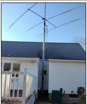
Complete crank up tower assy with tribander yagi, rotator, all located in Chicopee, MA. Being sold by Pete Kandilakis, KC1RY. Asking \$500
