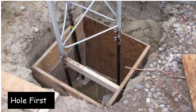
Leveling the first tower section before pouring
