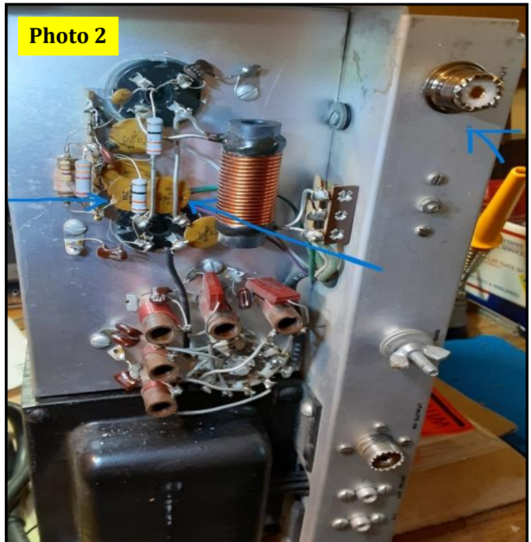
Cracked ceramic disk capacitor and SO-239 socket. Credit: B. Cook
